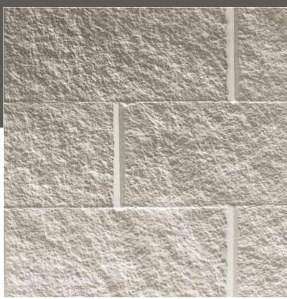
Liners have match-lines through blocks at vertical liner sheet seams.
