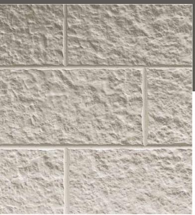
Liners have match-lines through blocks at vertical liner sheet seams
