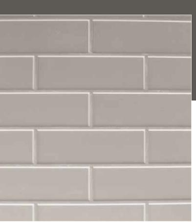
Liners have match-lines through bricks at vertical liner sheet seams.
